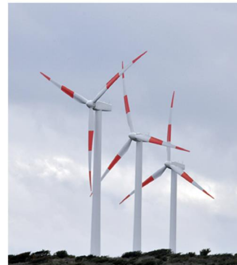
Wind park Cabo Negro: Power 2,5 MW (operating since 2015)
