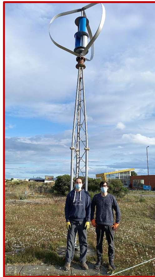
Wind generator VAWT, 700W
